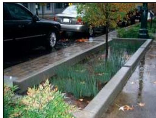
Open and closed drainage - this bioretention swale (open) treats sidewalk runoff before it is directed into the storm water system (closed). Photo: Nevue Ngan Associates - [www.gradingandexcavation.com/sw\\_0701\\_integrating.html](http://www.gradingandexcavation.com/sw_0701_integrating.html)
